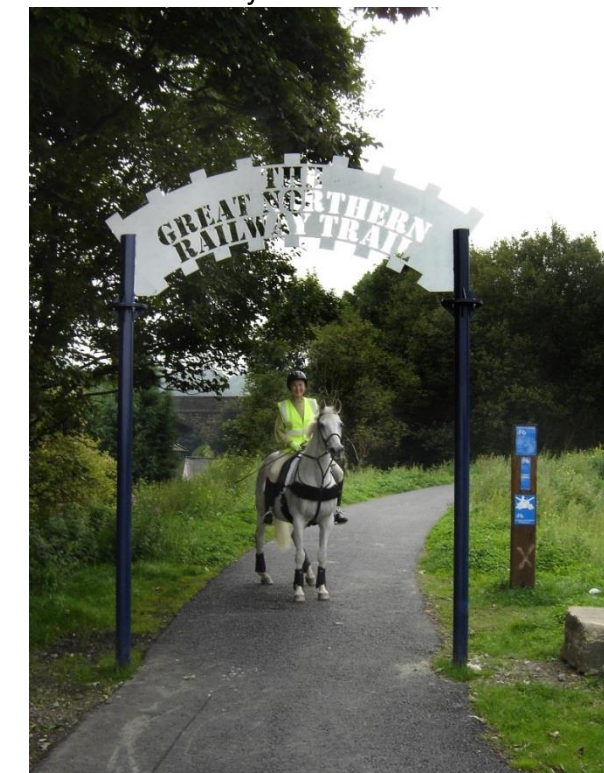
Formal access can be used to create Track 'gateways'; there needs to be enough headroom for all users as shown in this example from The Great Northern Railway Trail.
